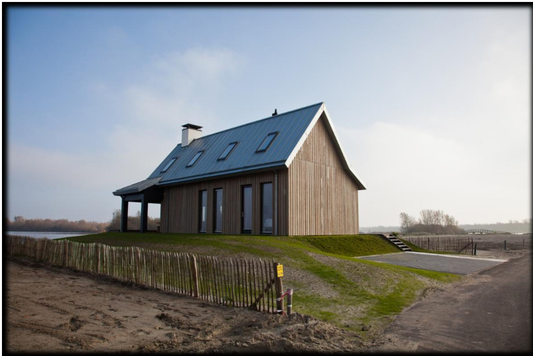
New House on mound to avoid damage in case of higher water levels in Lake Volkerak – Zoom – The Netherlands. Source: Ms. Ir. Loes de Jong
